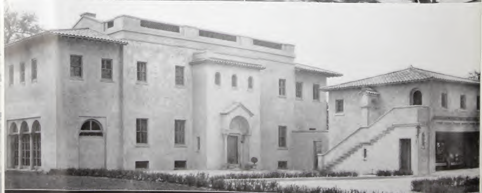
(Top) Masonic Home, Wichita, Kan. Tilton & Gihens, Architects, New York, N. Y. General Contractors, The George H. Siedhoff Construction Co., Wichita. Both Medusa White and Gray Waterproofed Cements used in the stucco.
